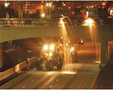
*"Washington Street Bridge – removing metal railing prior to structure demolition*
