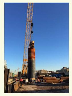
Driving 10' diameter casing for new eastbound structure
