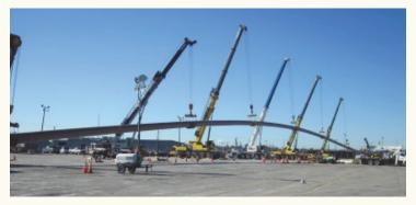
The 4,500 linear ft. subaqueous section of the new 36-in. water main was assembled on the Portsmouth side of the river and installed in one weekend, minimizing impact to the public
