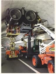
New jet fans installed in the existing tunnels are an upgrade to meet current NFPA fire life safety requirements
