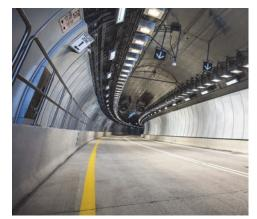
The tunnel ventilation utilizes a ceiling-mounted longitudinal jet fan system with reversible flow capabilities to clear smoke and heat away from
