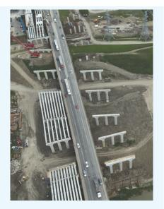
"Outside-In" construction allowed the existing roadways and bridges to remain in service during construction
