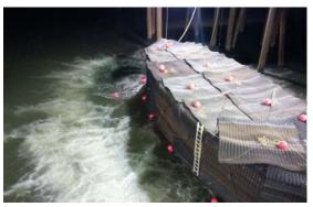
Kiewit implemented bubble curtains, fish deterrents, and comprehensive monitoring to protect aquatic wildlife during the demolition of large piers on the existing Port Mann bridge
