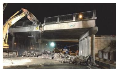
Gaglardi overpass entailed full demolition and replacement. This operation required high levels of coordination, notice, closures, and planning to complete in just three days.
