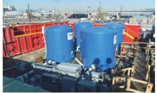
Treatment system for handling the contaminated dewatering
