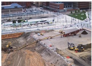
Conveyor system used for mass excavation work behind DUS
