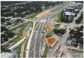
Construction first on the outside existing lanes minimized impacts to traffic
