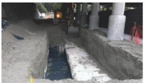
Ground improvements beneath First Avenue adjacent to existing columns were designed to account for local seismic activity
