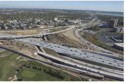
*I-25/I-225 interchange being constructed in phases to minimize impact to traffic*
